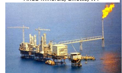
Offshore Gas Plant, Ardjuna Field ARCO Indonesia
