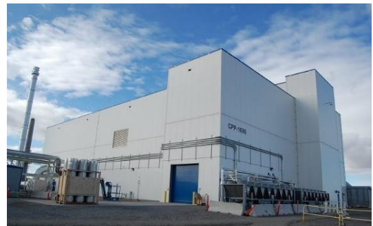
Integrated Waste Treatment Unit (IWTU) US DOE INL Site
